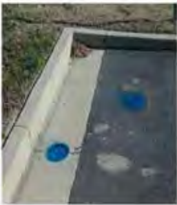
Valve box cover marking
