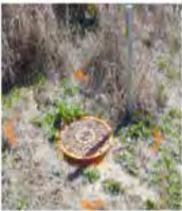
Manhole perimeter marking
