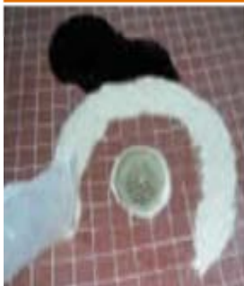
Floor Drains: use booms or drain covers to prevent oil from entering drains.
