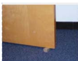
Fire doors should never be propped open by using a foreign object
