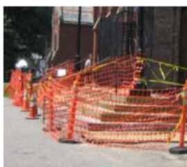
Blocked off construction site, creating a safety buffer for the public
