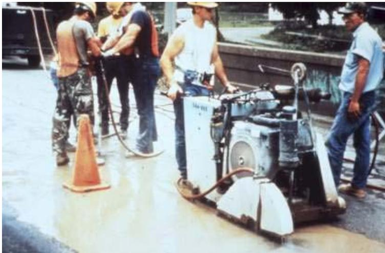
**Using water to cut concrete and bricks**
