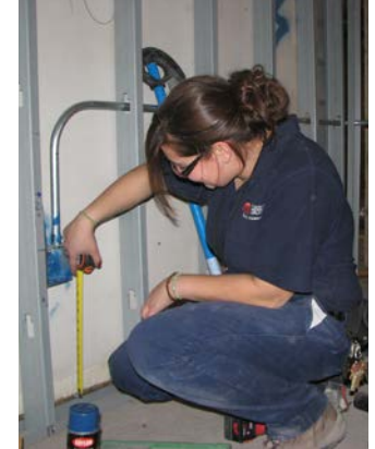
Electrician Apprentice Nicola Lemmer measures placement of receptacle boxes.
