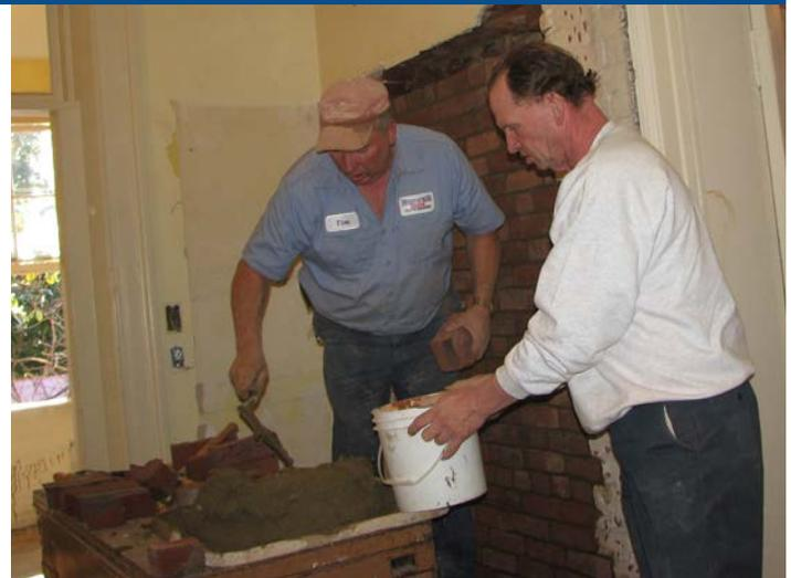
As the workday draws to a close, Masons Tim Proffitt and Glenn Tolbert work quickly with a new batch of mortar, filling in where a door was punched through an original wall.
