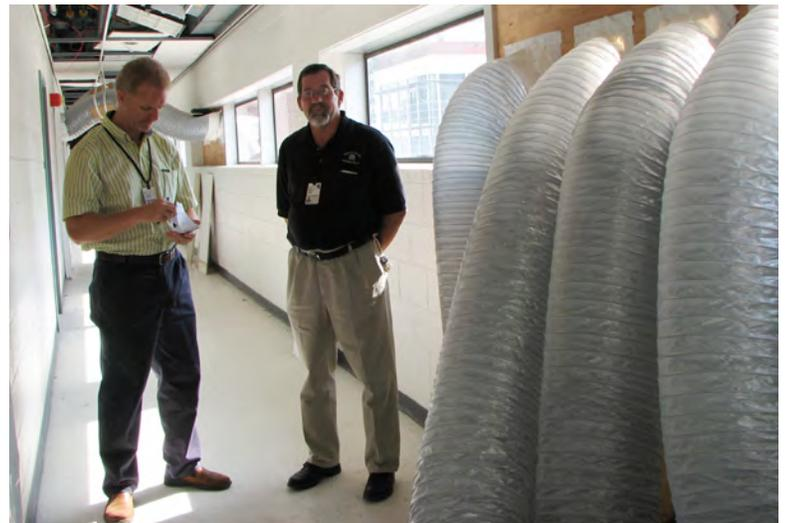
HSPP Work Management Supervisors Randy Speight (L) and Warren Britts review scheduling and inspect progress on the Old Jordan Hall fan coil replacement project. The large tubes on the right are in place to remove construction dust from the staging room where materials are adapted, cut and stored prior to installation.
