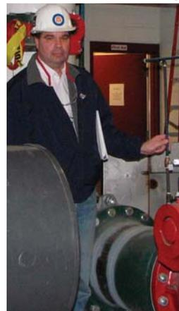
pumping system installation to one of the three 7000 gallon-per-minute secondary pumps. Construction Administration Manager Charlie Durrer explains the secondary pumping system to
