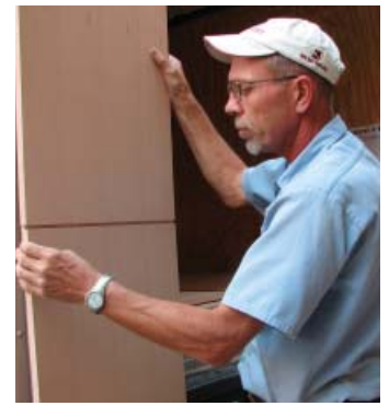
Darryl Napier checks the interlocking panel for hallways.
