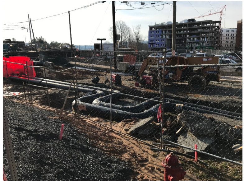
LTHW install in the new South Lawn Access Rd
