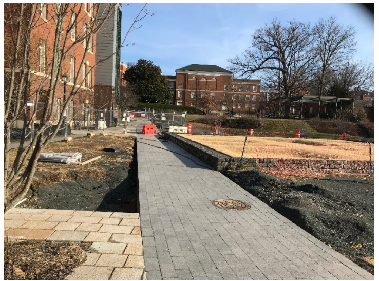
Reinstalled asphalt pavers at South Lawn
