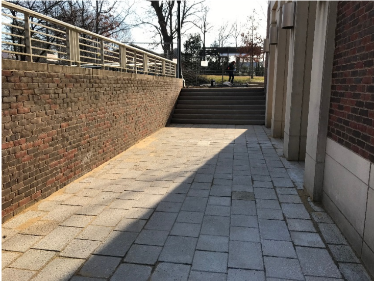
Reinstalled concrete pavers at South Lawn
