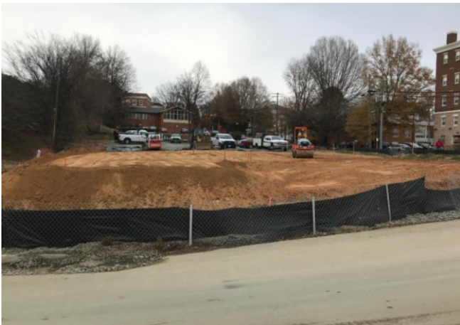
5. Construction of temporary access road at the 400 Blk
