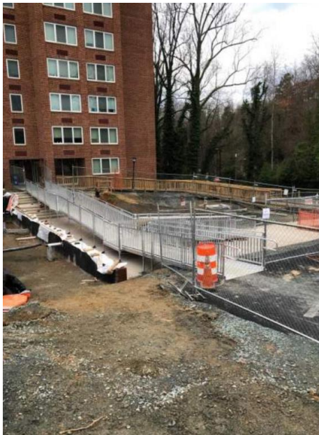
3. New ADA Access Ramp at Bice House
