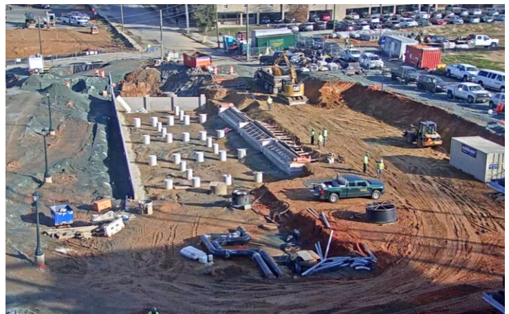
6. View of the bio-retention construction in lower Green Street
