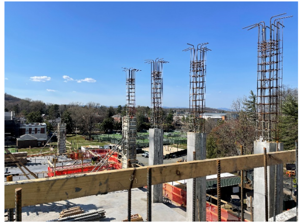
Rebar ready for Level 5 column forms
