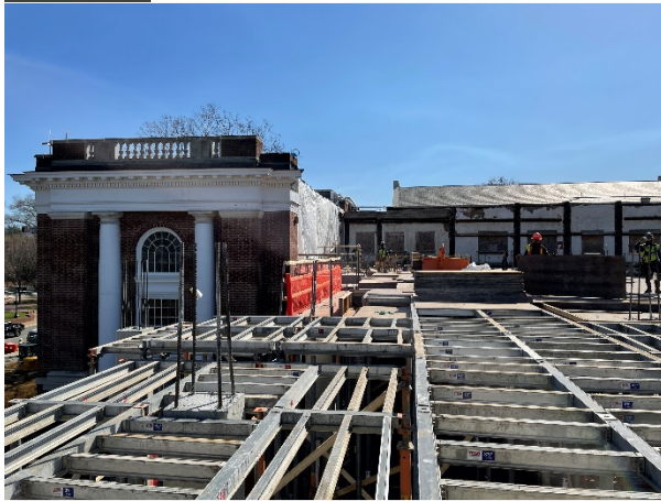
Decking formwork for Level 5 floor slab
