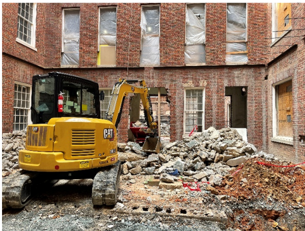
Future courtyard: slab demo, second floor windows converted to doors, bracing steel has been removed on level 1 and level 2.
