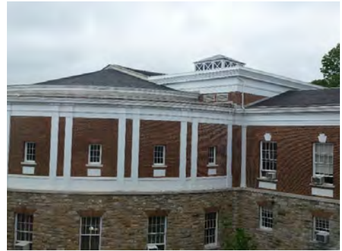
Old Cabell Hall This multi-faceted roof project will replace 15,300 SF of low-slope EPDM, steep-slope slate shingles, and flat-lock metal roofs along with all built-in gutters for a construction value of $1,035,000.
