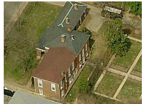
Hotel E Annex This roof project will replace 2,000 SF of steep-slope standing-seam metal with terne-coated copper. All gutters will be replaced, and metal flashing and slate repair will be performed on the Hotel proper. The estimated construction value for this project is $125,000.
