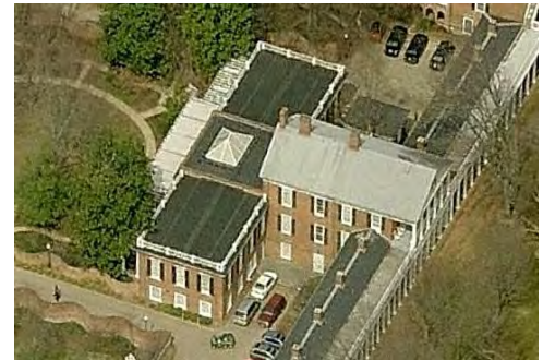
Pavilion VII The existing 4,300 SF low-slope EPDM roof will be replaced with a new fully-adhered EPDM roof at an estimated construction value of $145,000.
