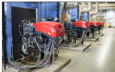
Utilities Supervisor David Hermes (top) was one of about 20 employees that assisted with a December project to install a temporary boiler at the Heat Plant; the Massie Road Plant's new high-efficiency and low nitrogen oxide burners (bottom) contributed to reducing the plant's nitrogen footprint.
