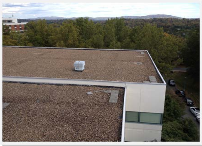
Withers-Brown – Roof before
