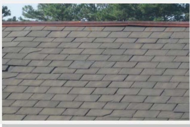
McIntire Wing – Roof before
