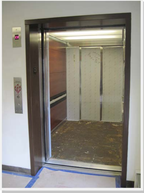
Thornton Hall E-wing - Modernization in progress
