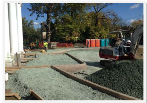
Rugby – Curb installation
