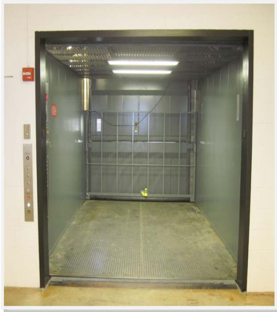
Mechanical Engineering Freight - Completed
