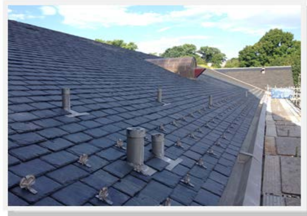
McIntire Wing – Roof after
