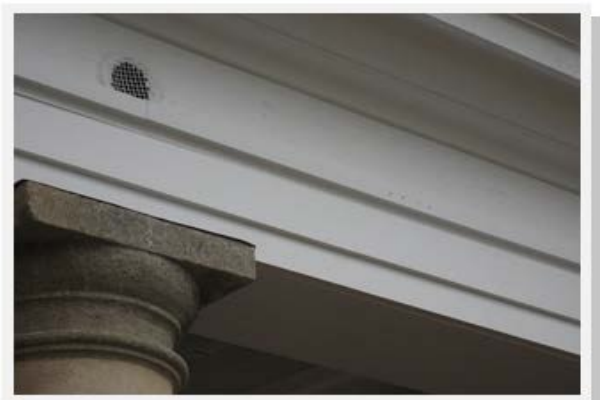
East Lawn – Colonnade support beam partial repair
