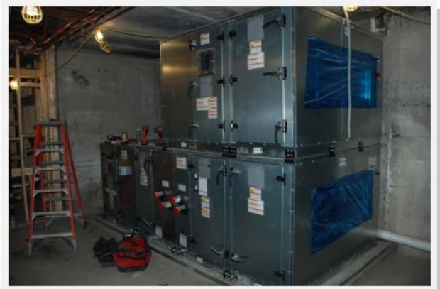
Rugby – New AHU in lower level mechanical room
