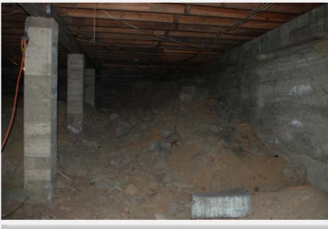
Rugby – Pool under main floor before
