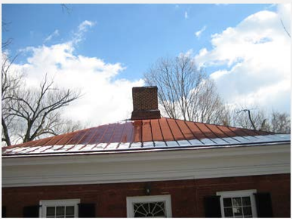
Hotel D – Roof before
