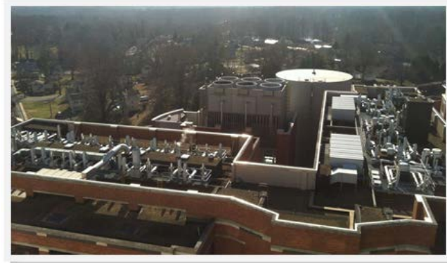
MR-4 – Roof before
