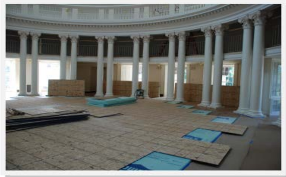
Rotunda – Dome room protective enclosures
