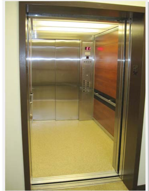
Thornton Hall E-wing - Modernization completed
