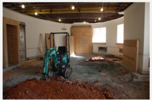
Rotunda – East oval room demolition of slab
