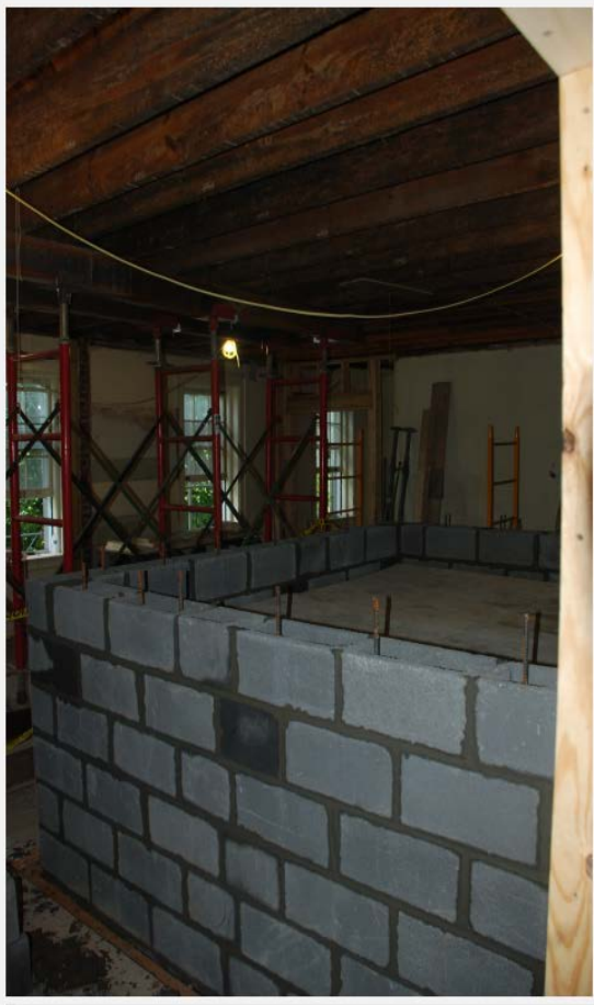
Rugby – Elevator shaft being constructed
