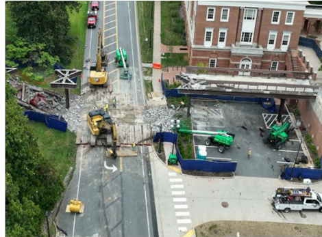
Ridley Bridge – Demo In-progress
