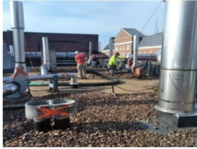
Med School Bldg – Roof Before
