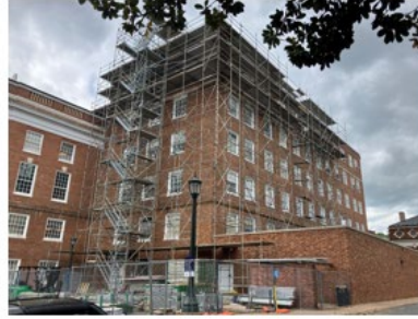
Med School Bldg – Roof In-Progress
