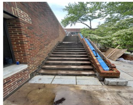
Clemons Library waterproofing– 80% complete
