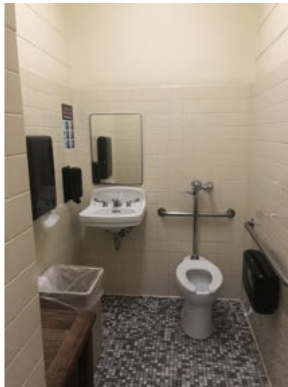
Thornton Hall – Bathrooms Before
