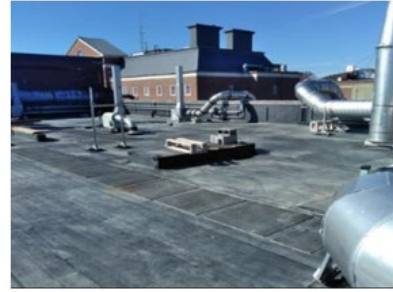
Med School Bldg – Roof After
