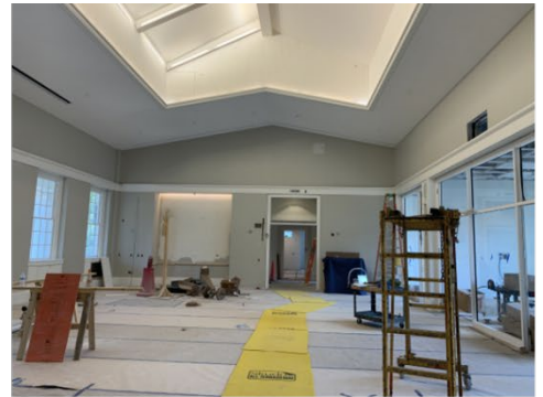
Cobb Hall – Interior Renovation In-Progress
