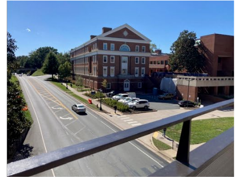
Ridley Bridge – After
