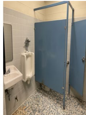
Thornton Hall – Bathrooms Before
