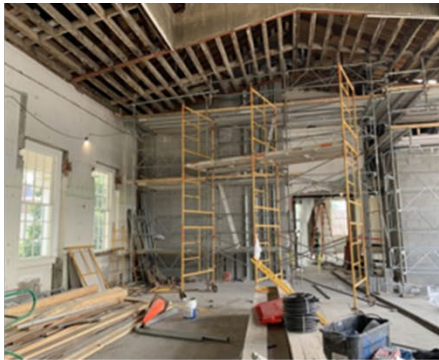
Cobb Hall – Interior Renovation In-Progress
