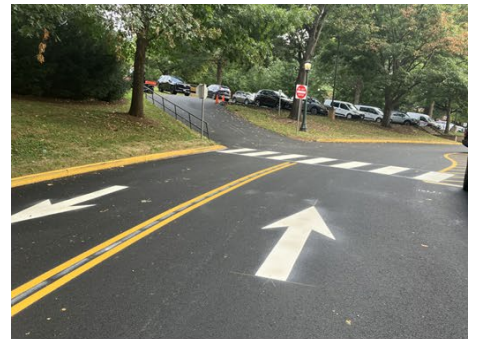
Hospital Dr – Road and markings after
