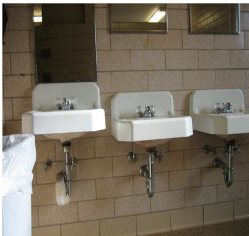
Kerchof Hall – Bathrooms - Before
