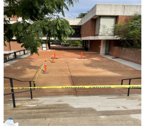
Campbell Hall Plaza Phase II – Complete
