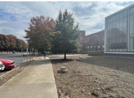
McCormick Rd – Sidewalk condition - Before
