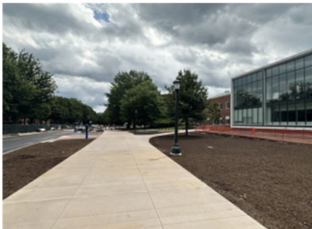
McCormick Rd – Sidewalk condition - After
