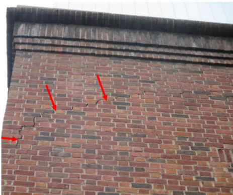
North Chiller Plant – West exterior wall - Before
