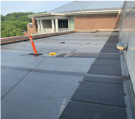
Chemistry Addition – New Roof
