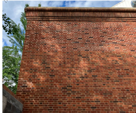
North Chiller Plant – West exterior wall - After
