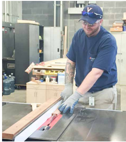
Project Services Cabinet Shop Supervisor Stu Fontaine (far left) reads blueprints for the casework/trim at the Darden Camp Library; Project Services Senior Cabinet Builder Brett Bryant (center) works on trimming panels for rails for the Pavilion V step repair project.
