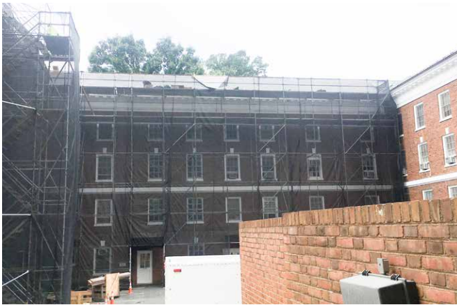
The re-roofing of McKim Hall's slate roof started in March 2017 with completion date scheduled for July 2017.
