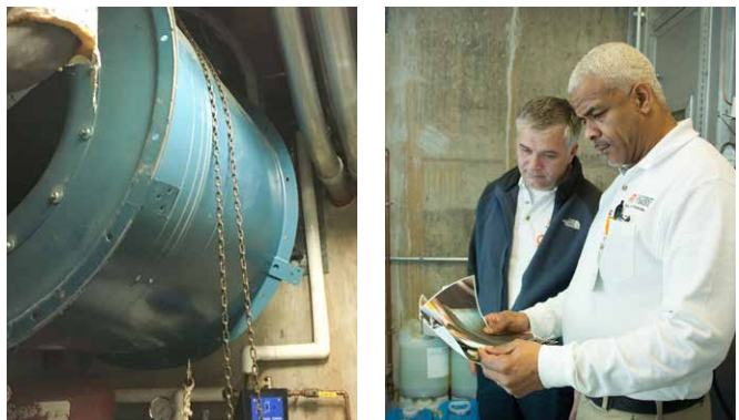
HSPM Zone 2 Superintendent Gary Allen and Zone Maintenance Supervisor Jake Bajs helped develop an innovative way to repair an exhaust fan in Pinn Hall by using a pulley system instead of installing scaffolding.
