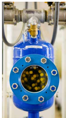
The Chiller Plants support sustainability goals with several projects, including a new medium temperature hot water converter in the Chemistry building (left); and the use of condenser tube cleaning systems (right).
