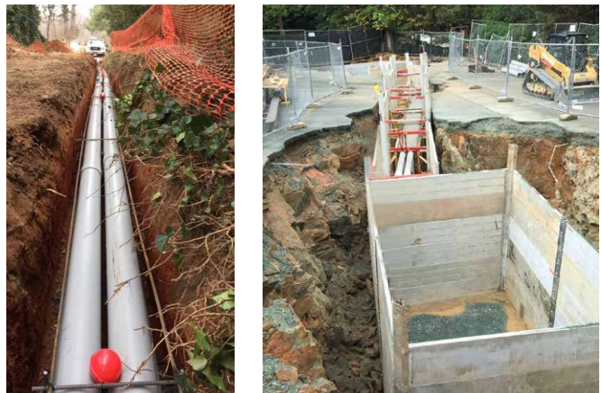
The Power & Light team self-performed the extension of the Davenport Stadium ductbank (left) in early 2017. The team continues to support and project manage the ongoing 35kV electrical ductbank project (right) which will construct an almost three mile underground power feed to UVA connecting three existing substations (Sherwood, Alderman and Cavalier).
