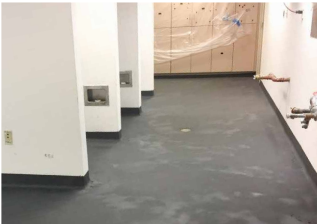
The Digestive Health Endoscopy renovation included new walls, monolithic poured floors and cabinets.
