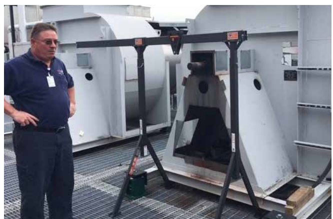
HSPM Zone 2 Zone Maintenance Supervisor Brian Gibson (pictured) and HVAC Installation and Repair Technician Senior Zeke Matic replaced an 800-pound exhaust fan motor on the rooftop of Pinn Hall.
