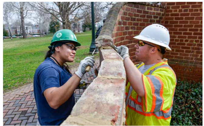
Project Services Masons (left photo from left) Lance Rothgeb and Timmy Proffitt prepare historic fabric for the new porch at the Colonnade Club as part of the Pavilion VII Porch Renovation project; Project Services staff (right photo from left) Mason Daisy Maine and Mason Apprentice Shane Harris carefully patch a brick section of a serpentine wall.
