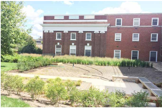
Re-roofing projects over the past fiscal year included the replacement of an underground roof for the Urology Department which was started in October 2015 and completed in November 2016. The underground roof, located off Hospital Drive, is covered with plantings and bench seating.
