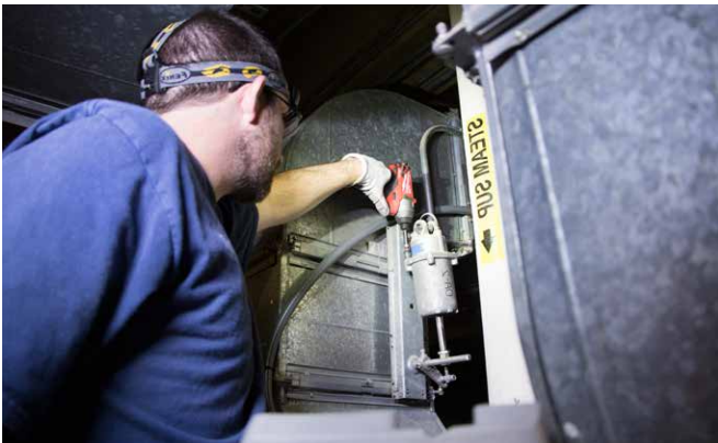
Delta Force has completed multiple projects to reduce energy use in buildings, including Newcomb Hall. Automation Services HVAC Apprentice Casey Morris removes old pneumatic controls which were replaced by new electronic controls in the building.
