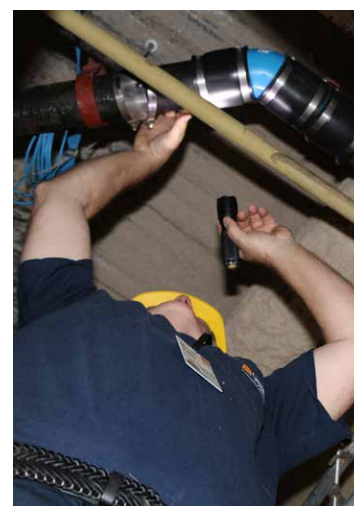
HSPP Zone 1 Plumber Assistant Matt Todd, left, and Plumber Steamfitter Chuck Kritner quickly fixed the cast iron fittings on a pipe that was leaking above the ceiling in the University Hospital.
