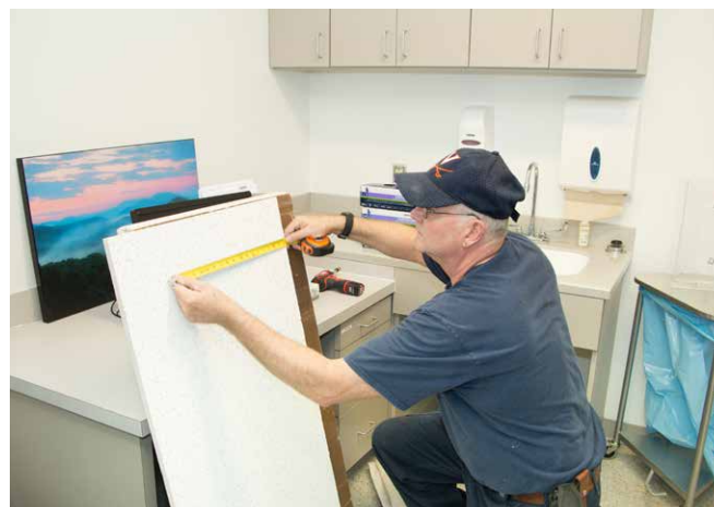
HSPP Zone 3 Carpenter Eddie Dodd replaces a ceiling tile after plumbers fixed a burst pipe.
