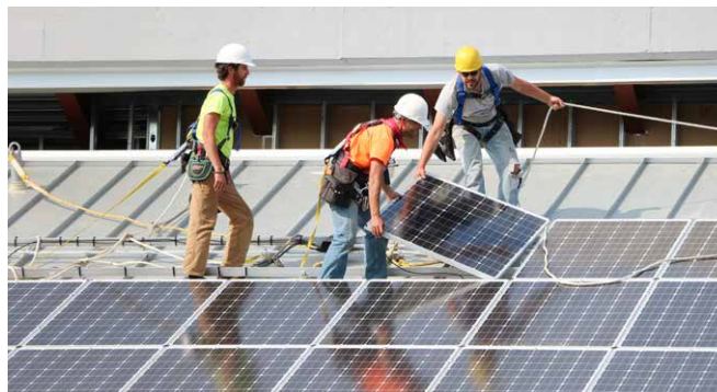
Workers with contractor Altenergy Inc. install a 15-kilowatt solar panel system atop Skipwith Hall in October 2015. This project was the first major solar panel installation at the University, with plans for larger projects in the near future.
