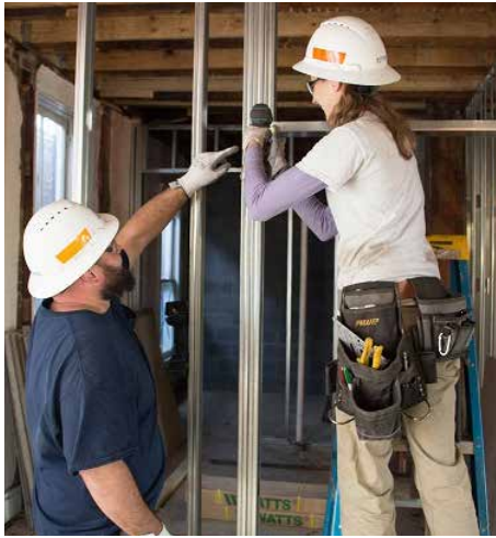
Carpenter Mark Lamonds and Carpenter Apprentice Anne Tufts install metal studs on the second floor of the 1515 University Ave. Student Center.
