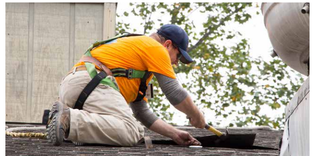
Volunteers included, from left, Custodial Services Worker Kiteto Mukala scrubbing a shower in a cabin; Housekeeping Supervisor John Carey dusting lights in the Dining Hall; and Roofer Glenn White, installing a tie-off hook on the Dining Hall roof to ensure roof maintenance can be performed in safer manner.
