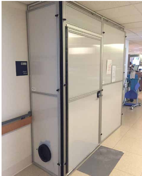
These partitions are one of the Infection Control Techniques used within the University Hospital when construction and renovation occurs adjacent to patient care areas.
