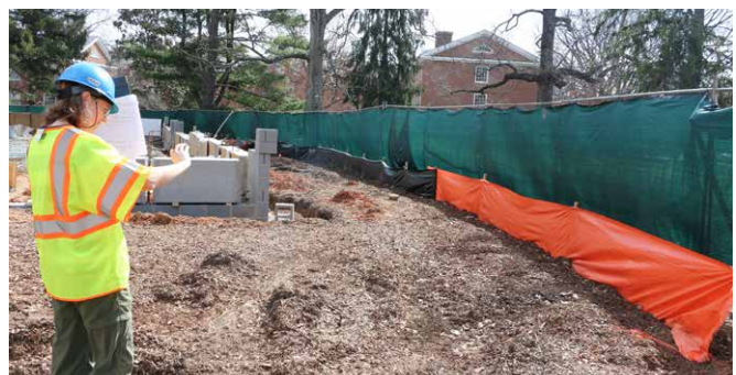
Environmental Resources Environmental Engineer Kristin Carter captures photos of an erosion control fence on the Cemetery Expansion site. The team conducted 341 individual erosion and sediment control inspections of UVA projects during the past fiscal year.
