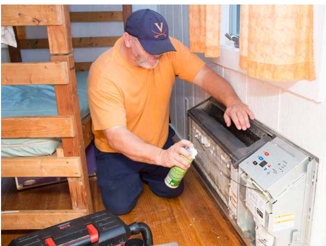
HVAC Mechanic Frankie Henshaw cleans an air conditioning unit coil in a Camp Holiday Trails cabin.
