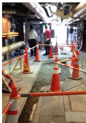
A new brine pipe trench (left) installed earlier this year at the Heat Plant will prevent future deterioration of the condensate system. Heat Plant Boiler Operator Danielle Borgus (right) tests the water that will be used by the boilers to ensure it is the proper pH.
