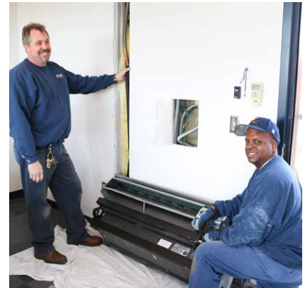
West Grounds Maintenance staff upgrading suites at Davenport Field to include air conditioning, included, Plumbing Apprentice Kristina Williams, left, installing new pipe in the concession area to tie into the suites above and HVAC Senior Mechanic Beau Ludovissy and HVAC Assistant Corey Harmon installing the AC unit inside the suite.
