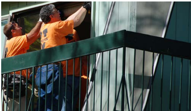
At Camp Holiday Trails Project Services Carpenter Matt Pannell and Review Unit Managing Architect/Engineer Bob Waite removed a sliding glass door and the frame so they could repair the floor that had rotted out.
