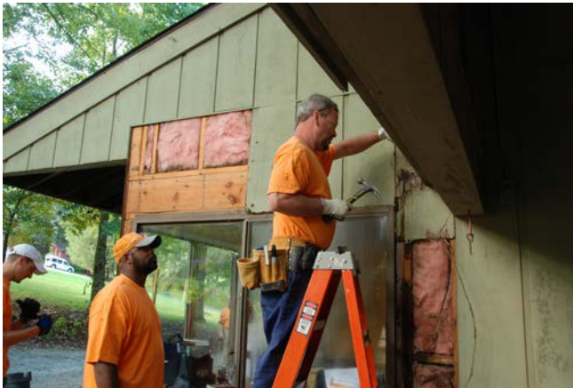
Information Systems' Jacob Neal and Keith Southerland, and Project Services' David Simpson replaced deteriorating exterior siding.
