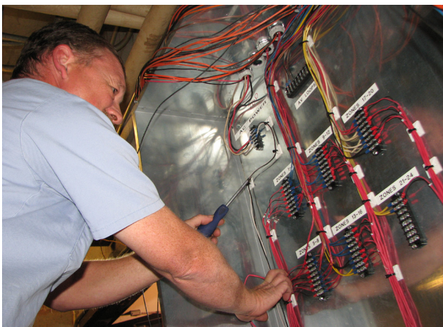
Electronics Apprentice Bobby Stanley makes adjustments for a fire panel installation.
