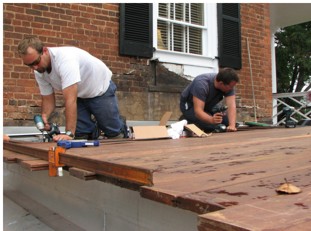
The Ipe wood that Carpenters Matt Pannell and Travis Sly are installing for the Colonnade roof replacement was chosen for its strength and resistance to weather and pests.
