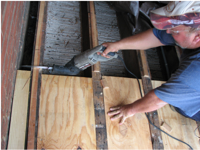
Lead Carpenter Walter Harris cuts the crosspieces to ensure a firm fit for the flat roof deck system over Lawn rooms 35-51.
