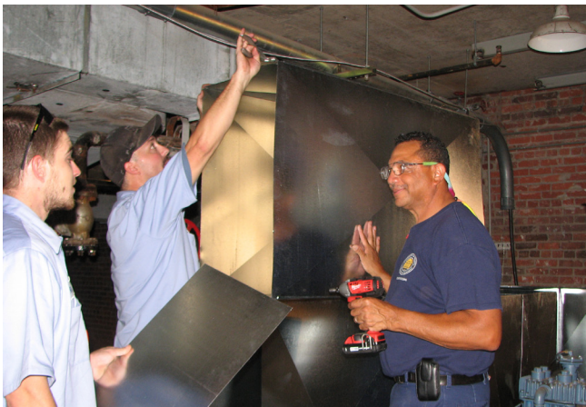
Sheet metal crew Robert Zakaib, Darrell Carr and Marcellus Dent complete ductwork for a new, more energy efficient HVAC system in Clark Hall.
