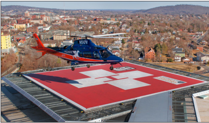
Photo by Jennifer Watson/FM Webmaster The UVa Medical Center Hospital Bed Expansion and Helipad Project — which was managed by Facilities Planning & Construction’s Health System Division — was named Best of the Best 2013: Best Healthcare Project by Engineering News Record in December 2013.
