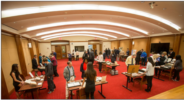
Photo by Sanjay Suchak/UVA Communications New energy-saving fluorescent lamps were recently installed in the Harrison Small Special Collections Library auditorium. The lamp replacement improved the efficiency and quality of the lighting while reducing maintenance costs.
