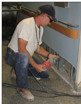
After a water pipe broke in the ceiling of University Hospital 6 West in August 2013, HSPP crews responded immediately, cleaning up and making repairs following the significant flooding in 5 and 6 West. Carpenter Lead Phil Kleinheinz (left) removed damaged sheetrock and insulation and Renovations Trades Utility Worker Maurice Gough (right) helped clear debris so repairs could be made efficiently and safely.
