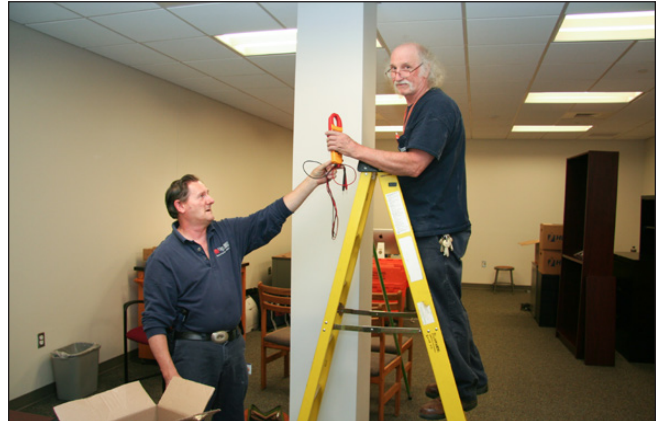
Maintenance teams often help departments settle into newly renovated facilities. Trades Utility Senior Worker Tony Thomas and Master Mechanic David Gentry finish utility work at Ruffner Hall, which recently underwent an 18-month renovation.
