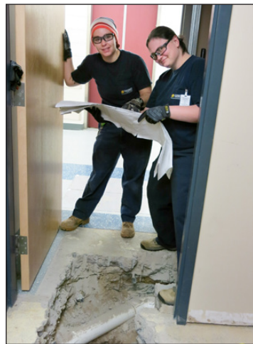
Plumber Steamfitter Mariah Kurpel, who graduated from the Apprenticeship Program in 2014, and Plumber Apprentice Kristina Williams look over drawings in preparation for a pipe repair during their rotation with Health System Physical Plant's renovations team.
