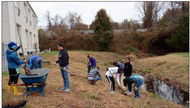
The Environmental Resources team worked closely with the Stormwater Task Force and the Materials Working Group of the UVA Environmental Impact Subcommittee on many projects, including installing new plants along a section of restored stream adjacent to Carr's Hill field.
