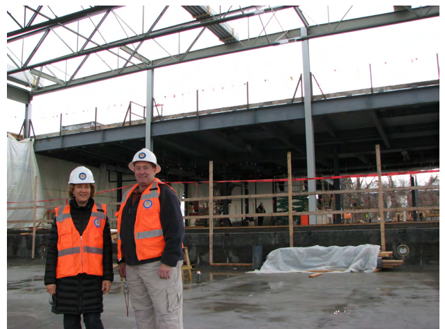
Earlier this Spring with construction well underway, Senior Project Manager Amy Eichenberger and Construction Administration Manager Charlie Durrer stand in front of the 10-lane pool in the North Grounds Recreation Center Expansion, the first of three planned projects to improve existing Intramural Recreational (IM Rec) facilities on University Grounds. The new 33,000 square foot addition, located to the west of the existing IM Rec Center building, will have an aquatics facility, a mind-body multi-purpose fitness room and two squash courts. Supervisory Senior Construction Administration Manager Steve Ratliff was unavailable for this photo. Completion of the new facility is scheduled for Fall 2013.
