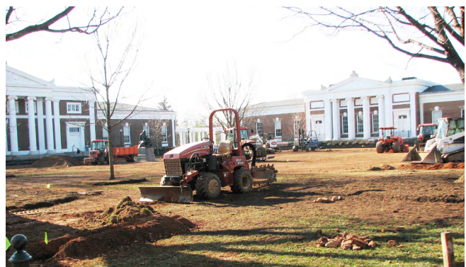
A full turf restoration of the South Lawn was the final phase of Landscape Division's unprecedented renovation of the Lawn.
