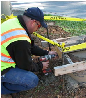
High Voltage Electrician Tim Gibson installs a new illuminated pedestrian crossing signal as part of the University's proactive concern for safety.
