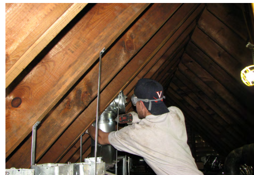
Sheet Metal Technician Robbie Zakaib installed custom designed ductwork made by the Facilities Management Sheet Metal Shop for the Dawson's Row renovation.
