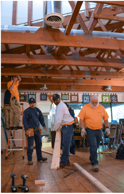
Left: In the Camp Dining Hall, a fleet of talented Facilities Management tradespeople built a new storage closet. Shown here are Kyle McCauley, Chad Simpson, Dillon Dean, Robbie Kincaid, Todd Stevens, Glen Marshall and Tommy Benson.
