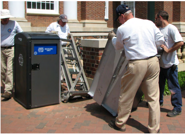
Landscape and Central Grounds Zone's Greg Rogers, Scott Burns, Donald Tooley and Chris Herndon joined forces to install a trash composter (BigBelly) and recycling unit (SmartBelly) outside Alderman Library in April. These two units, funded by Energy & Utilities and Operations & Maintenance, are part of a pilot project initiated by the University Committee on Sustainability to install solar powered trash composters and recycling containers which send real-time data to alert the Landscape Division office when collection is needed. The project addresses students' requests for more opportunities to recycle outdoors. The value proposition was that UVa could introduce more exterior recycling while requiring no additional effort from Landscape. A grant from Student Council's Green Initiatives Funding Tomorrow (GIFT) funded the first BigBelly/SmartBelly at Clark Hall.
